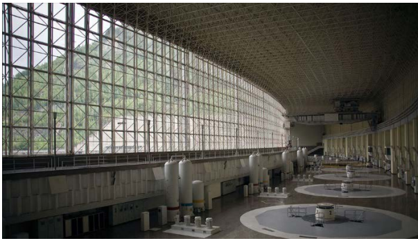
Figure 2: The Sayano–Shushenskaya hydroelectric power station before (left) and after (right) a catastrophic wreck of unit #2, one of its ten identical 640MW units. Root cause was traced to elevated vibration that fatigued the turbine’s mountings and head cover. 75 fatalities occurred as a result of this accident and estimated losses totaled $523M USD.
