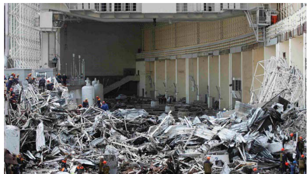
Figure 2: The Sayano–Shushenskaya hydroelectric power station before (left) and after (right) a catastrophic wreck of unit #2, one of its ten identical 640MW units. Root cause was traced to elevated vibration that fatigued the turbine’s mountings and head cover. 75 fatalities occurred as a result of this accident and estimated losses totaled $523M USD.
