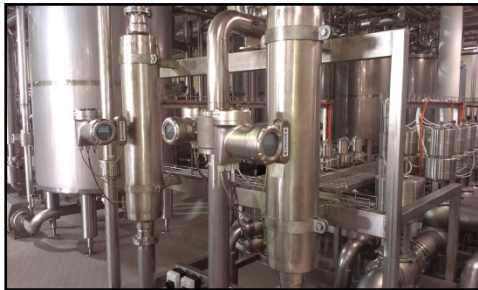
OPTIMASS includes entrained gas management system and provides full transfer with accuracy of 0.2 percent or less
