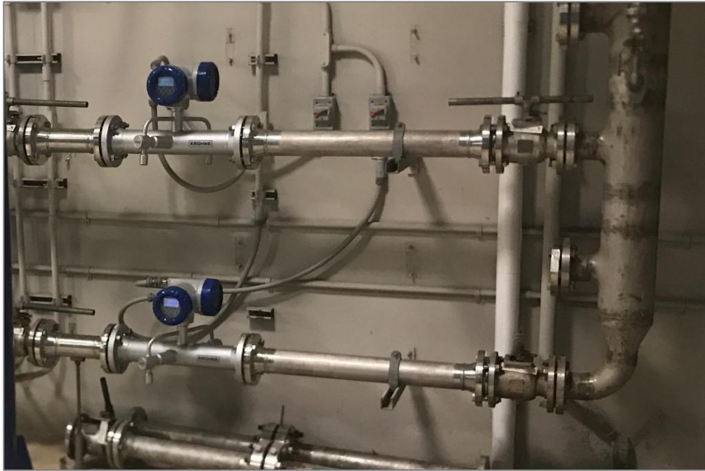
Figure 2 KROHNE OPTISONIC 7300C meters for Oxygen and Ozone gas flow applications
