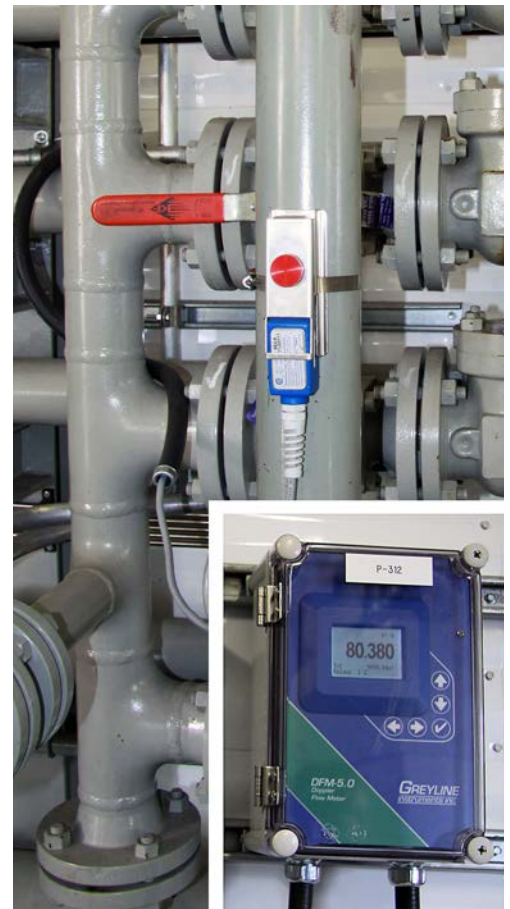
Left: Sand, Wax and Solids Removed in Crude Oil Treater. Below: Clamp-on Ultrasonic Transducer Monitoring Crude Oil Flow in 3" Steel Pipe
